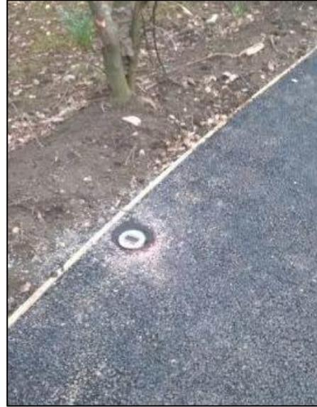
**Figure 12: New solar studs under trial**
