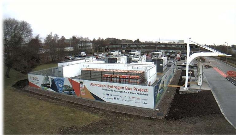
The refuelling station is consistently refuelling the buses in an average of 5 minutes, and has now completed over 1,600 refuellings.
